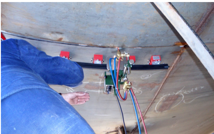
Overhead cutting made possible with strong permanent magnets
