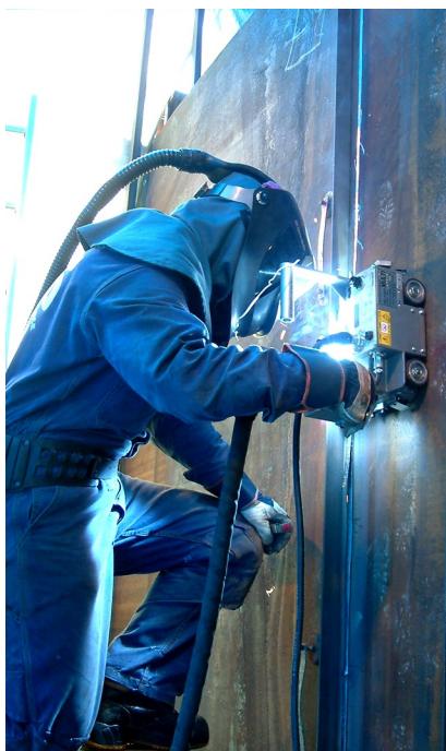
Vertical up butt welding using guide rail
